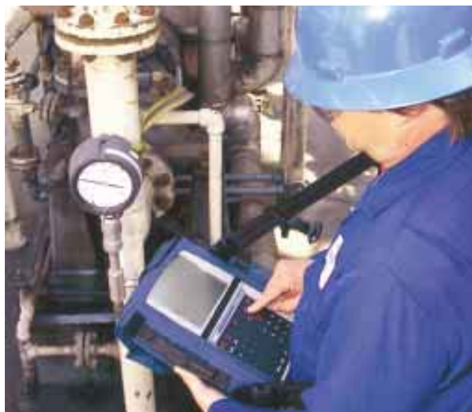
Microlog – portable data collector and analyser
