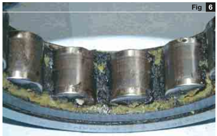
Black discoloured grease caused by passage of current
