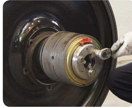
25 Tightening the end cap bolts
