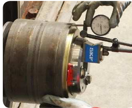
27 Installing the equipment to measure axial clearance in the tapered roller bearing unit
