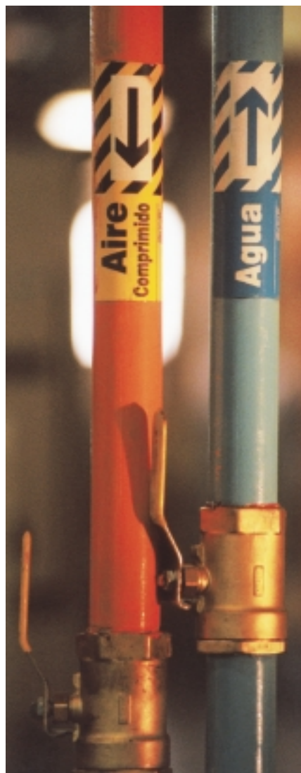
Figure 37 Pipework at SKF de Mexico, in Puebla is colour coded and labelled to ensure speedy identification in case of an emergency. The Service Business Unit at Puebla was one of 21 units to receive the SKF Zero Accidents Award in 2001.
