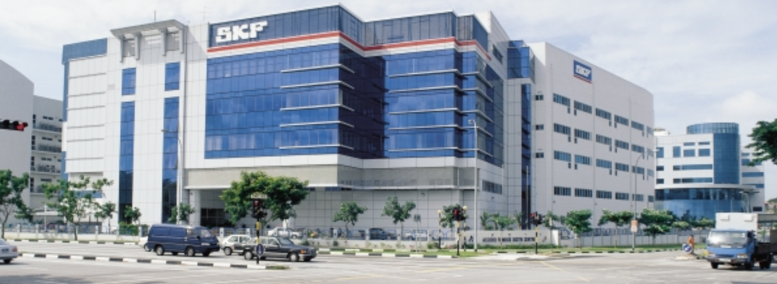
Figure 3 SKF's new Distribution Centre in Singapore achieved ISO 14001 certification in 2001. This approval was helped by the Centre's energy saving project, which cut electricity consumption by 22% compared with 2000.
