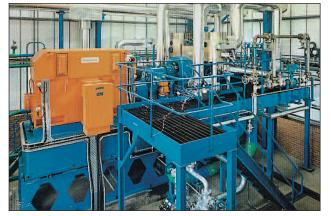
Steam Turbine Generator Set. Coupling fitted between the gearbox and alternator.
