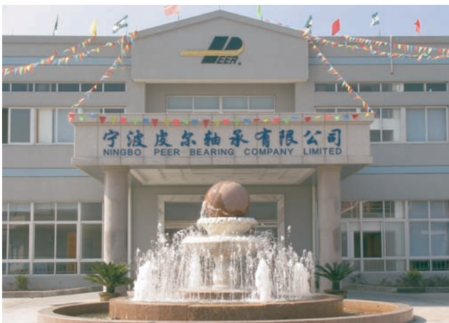
PEER Small Bore Bearing Factory, Cixi, Zhejiang, China
