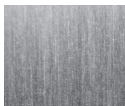
■ Good finished surface
