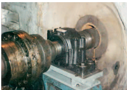
Bearing arrangements in fans and ventilators
