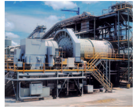
Bearing arrangements in comminution and processing plant
