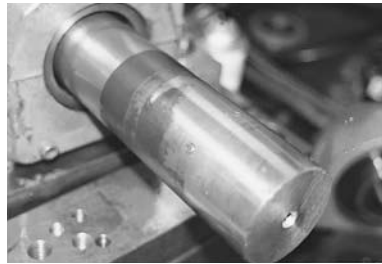
Typical fretting corrosion and shaft damage with setscrew bearing. Bearing quite often is "frozen" to shaft
